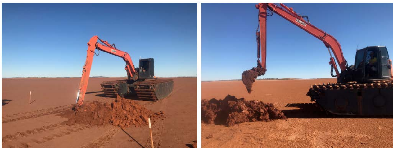
Figure 11: Amphibious Excavator on Lake Ballard
