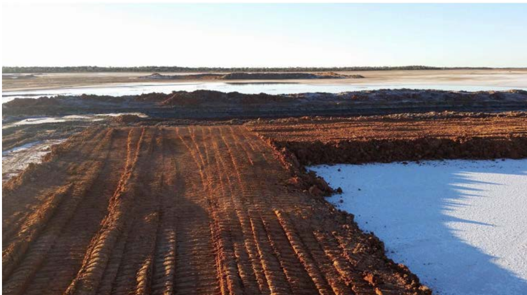
Figure 5: On-lake Evaporation Pond Construction at Lake Wells
