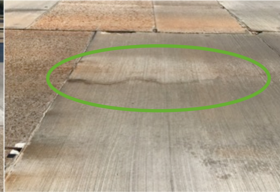
Control – Visible Crack Across Slab
