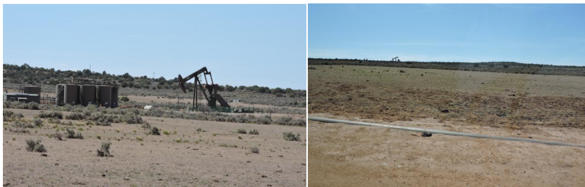
Figure 2: Photo of the oil pump jacks abutting the access tracks to the project area.
