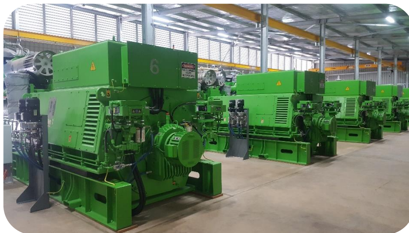
New Jenbacher 620 Spark Ignition gas generator sets installed at the Jundee Project
