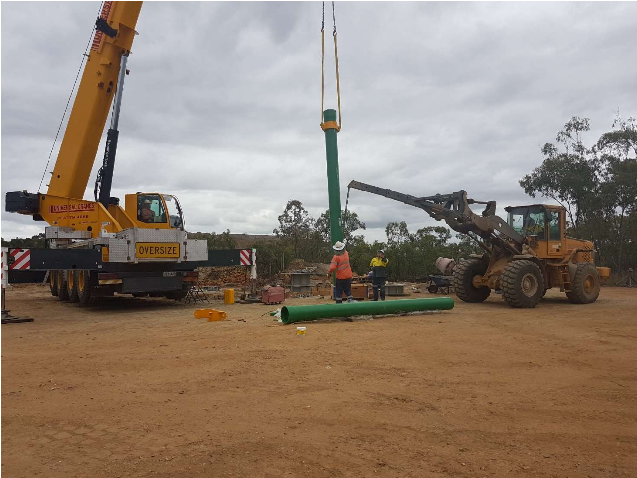
Installing the DRS dewatering bore at the Surveyor Project, July 2017
