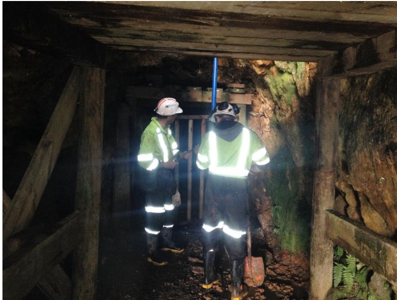
Figure 1 - Work in progress with support upgrades at the Talisman Project
