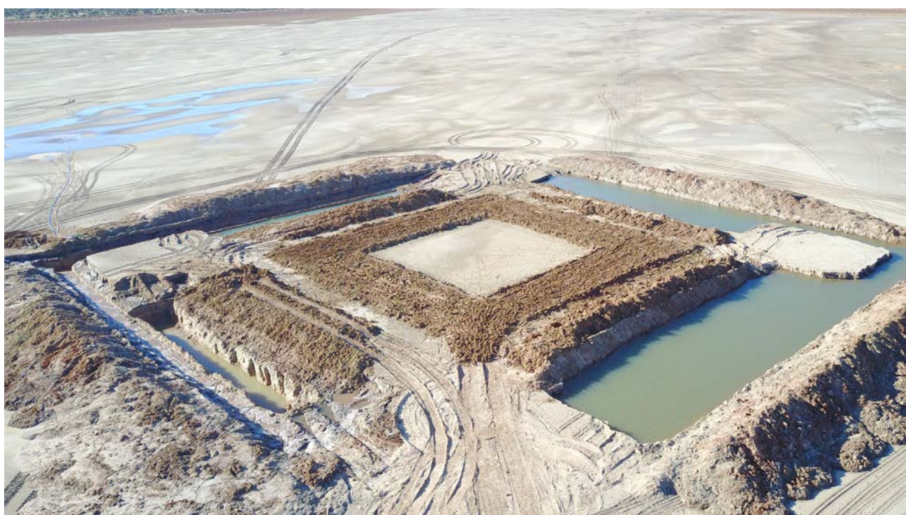
Figure 3: Construction of Evaporation Ponds on Lake Wells
