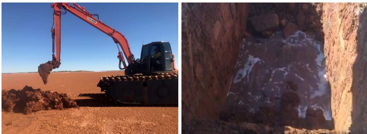
Figure 8: Amphibious Excavator on Lake Ballard and An Example Test Pit with High Flow
