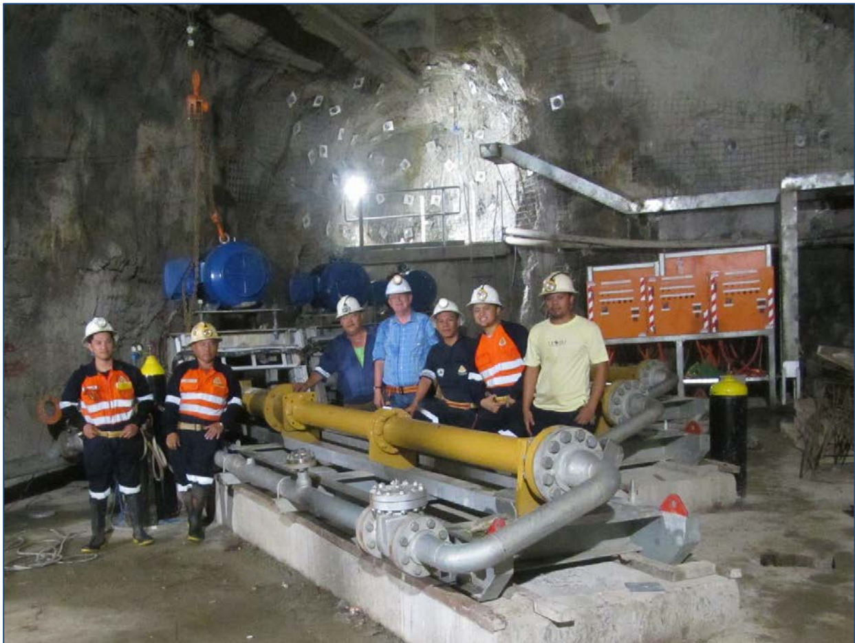
Figure 3: Construction team at level 8 pump station.
