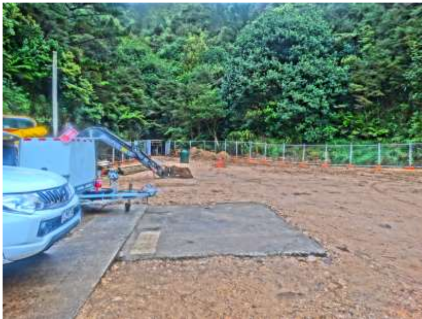
Figure 3- Portal pad as of July
