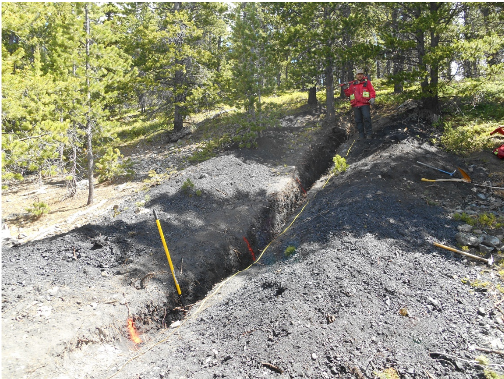
Figure 7: Trenching program at Elan Coking Coal Project
