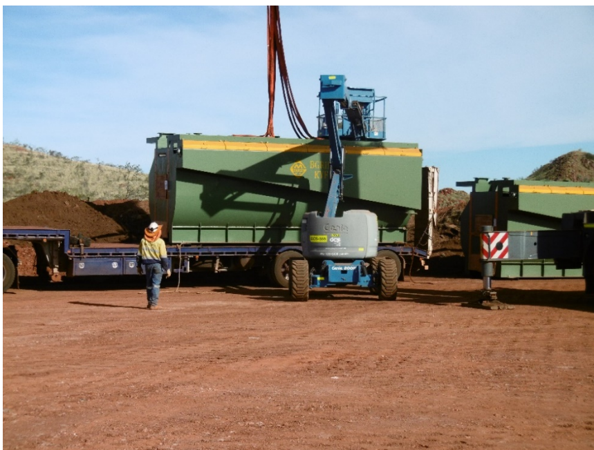
Flotation cells being unloaded on site
