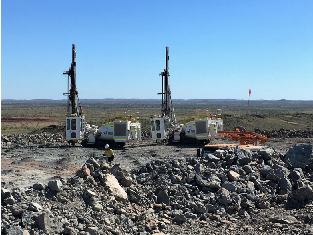
NRW drill rigs preparing for a blast in the pit
