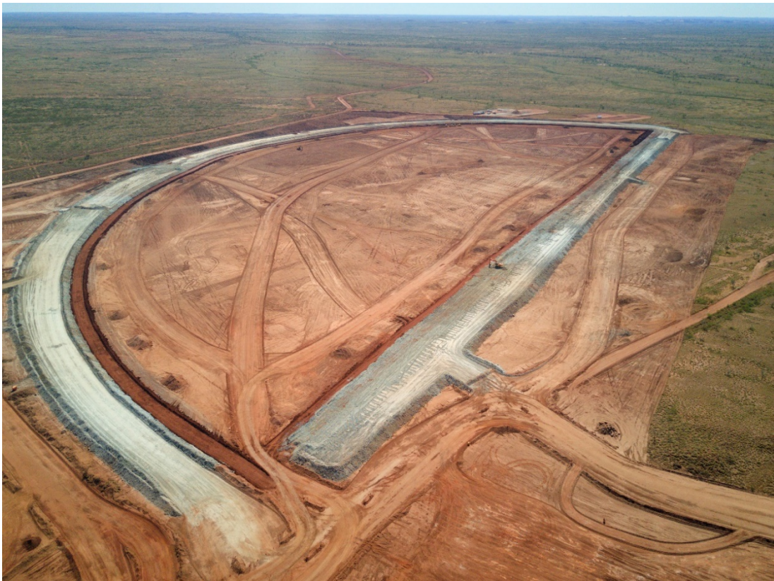
Tailings Storage Facility under construction
