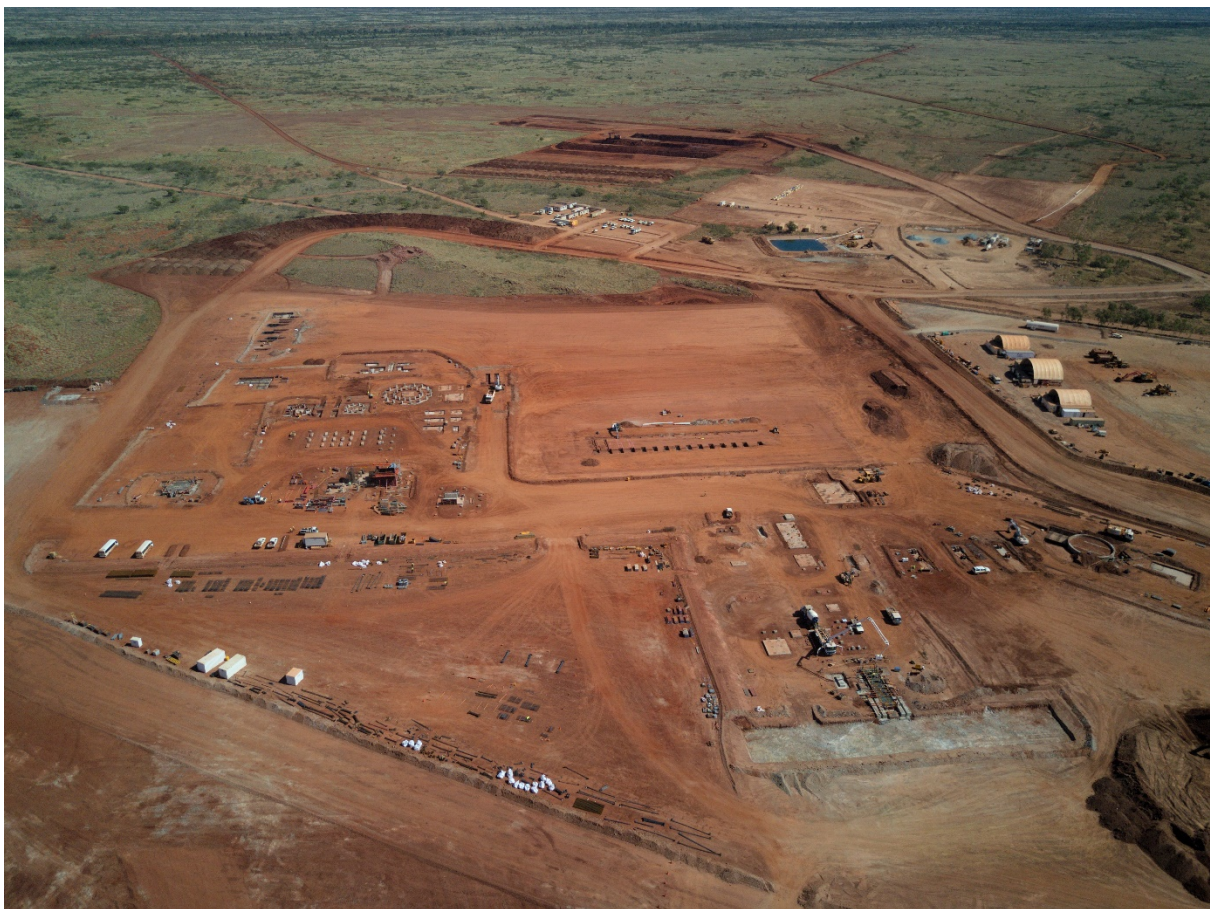
Progression of the concrete works for the process plant, looking west
