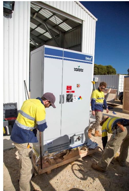
Delivery and install of Battery Energy Storage System (BESS) components
