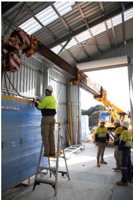
Delivery and install of Battery Energy Storage System (BESS) components
