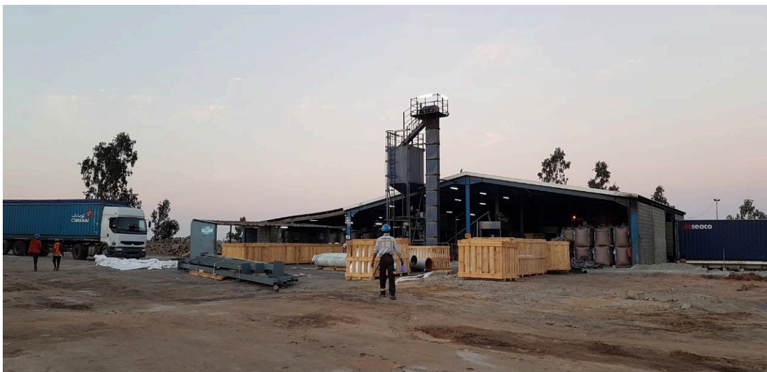
Figure 1: Unloading of the Modular Drying System components.
