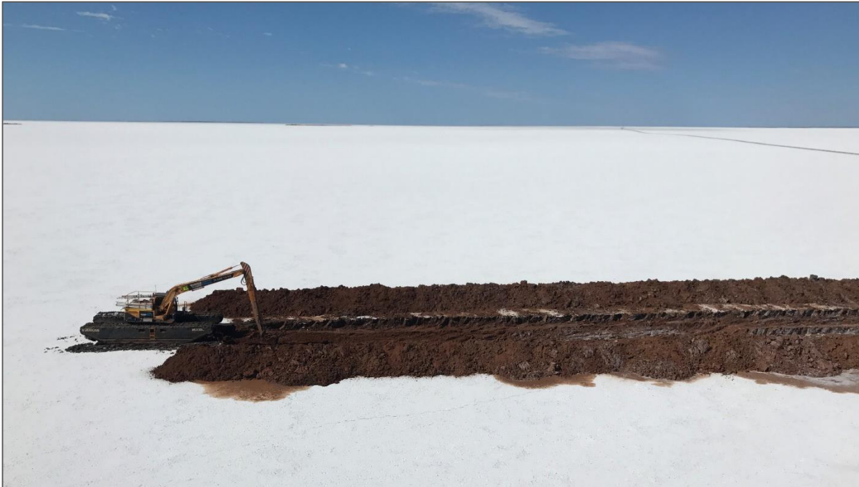
25 tonne Amphibious Excavator Currently on Lake Mackay
