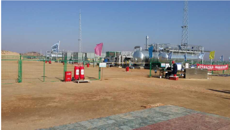
Sanjiaobei Central Gathering facilities commissioned
