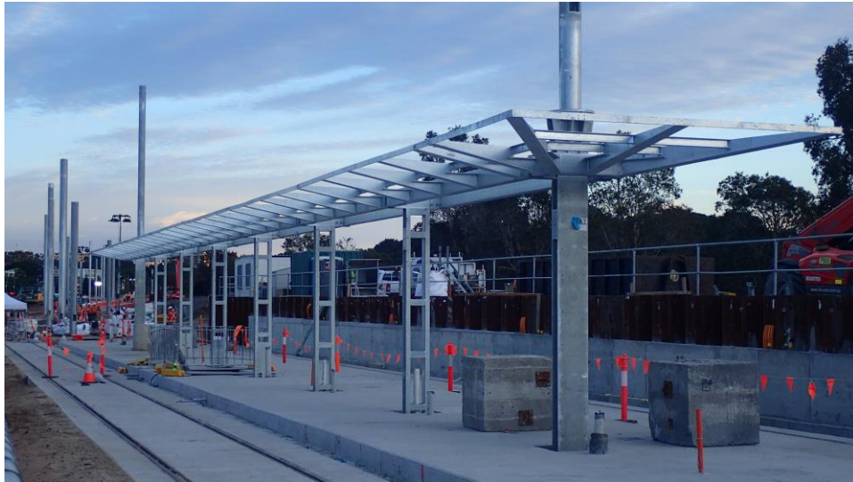
Sydney South Eastern Light Rail under construction (Randwick Racecourse Station) – 100% of exposed steelwork is galvanised
