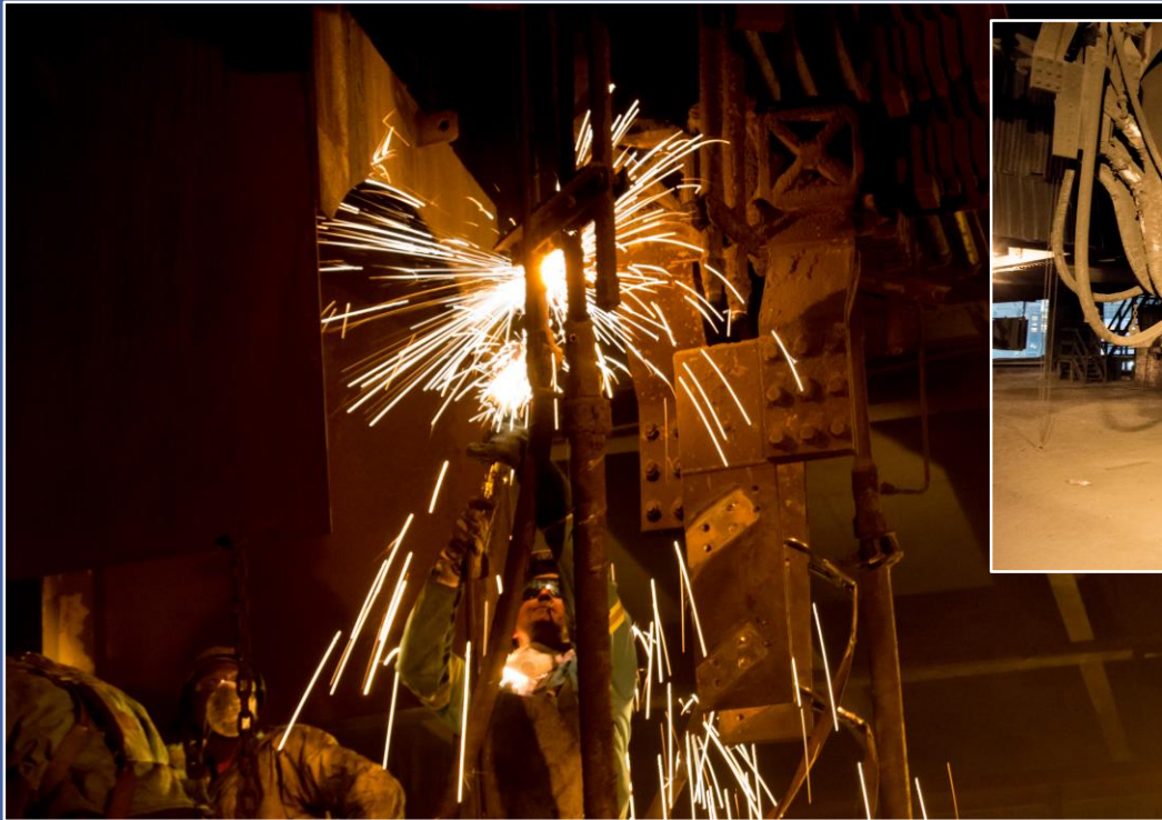
Smelter dismantling underway in South Africa
