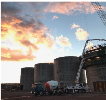
Bass Point Silos
