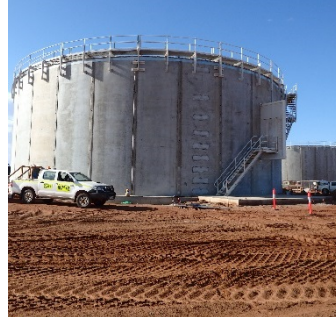
Onslow Water Tanks
