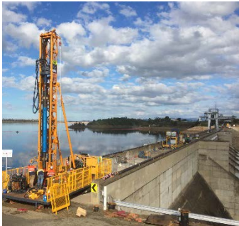
Keepit Dam NSW
