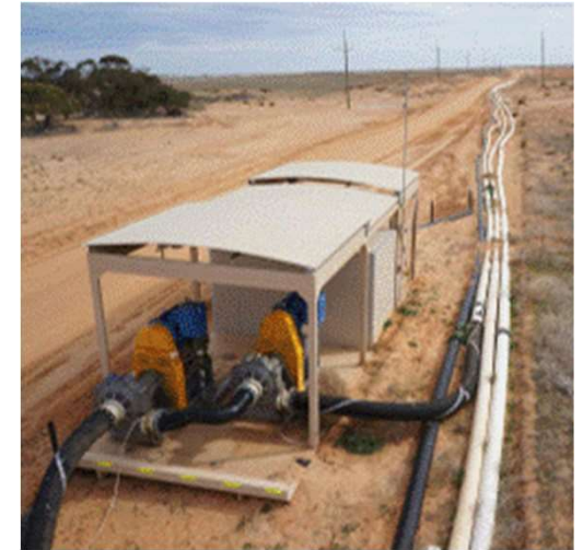
Slurry Booster Stations & pipelines
