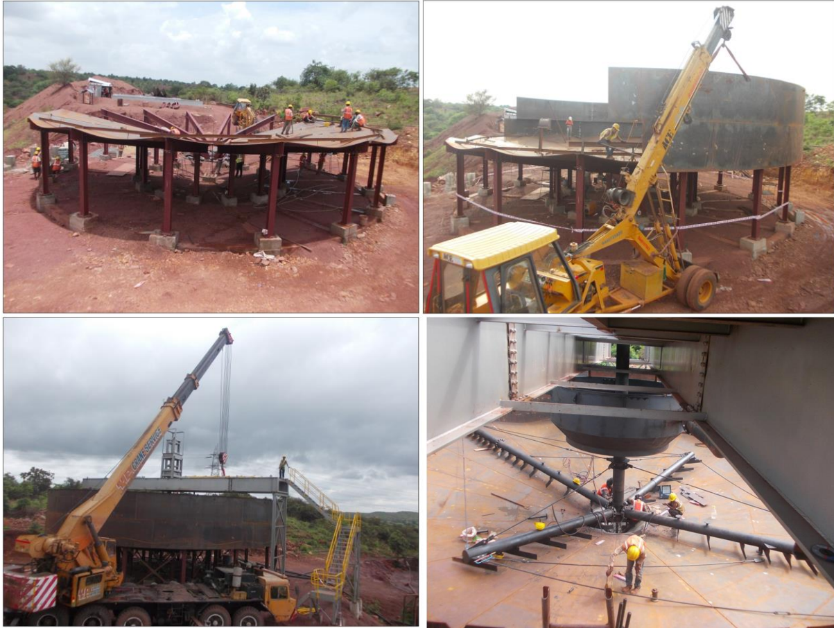
Thickener construction time lapse
