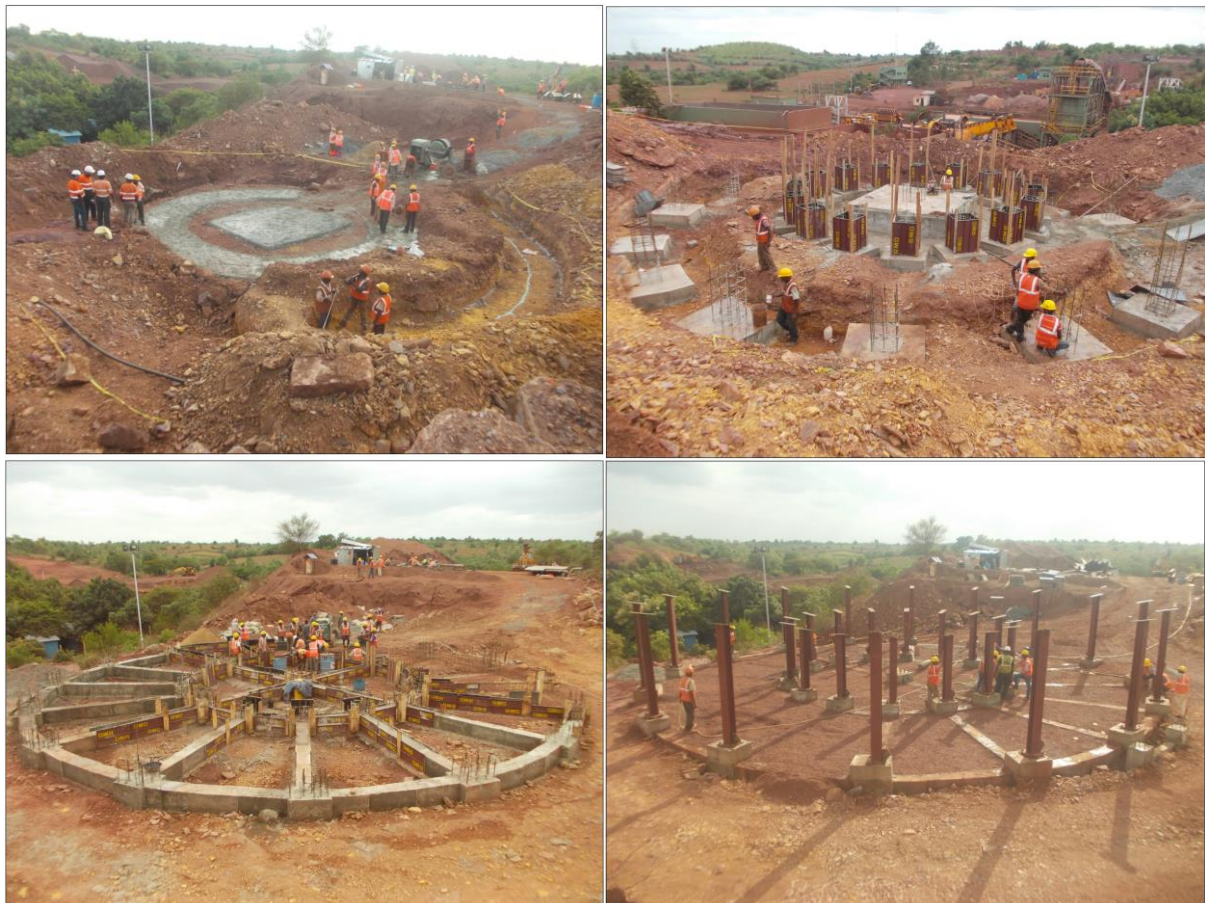
Thickener construction time lapse
