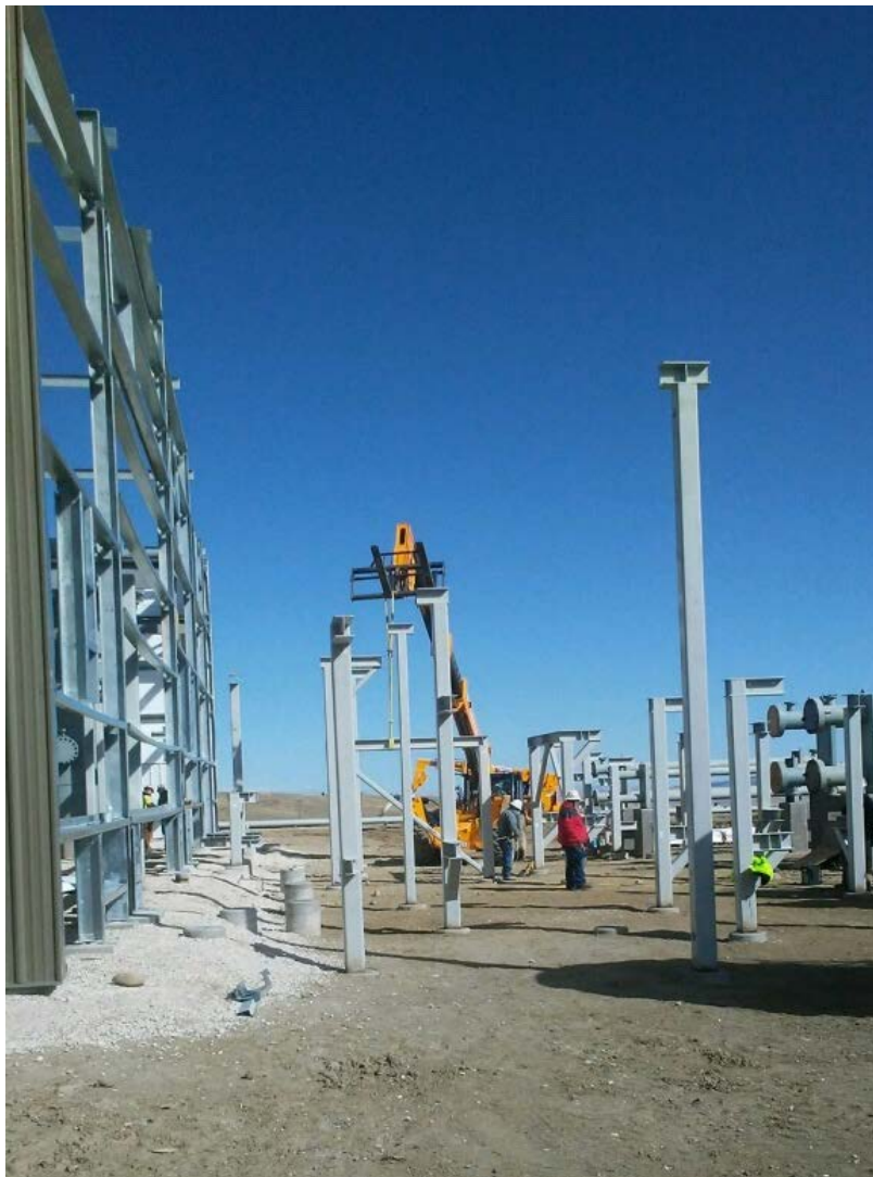
Compressor Building Piping Supports Being Installed – 22 September 2017
