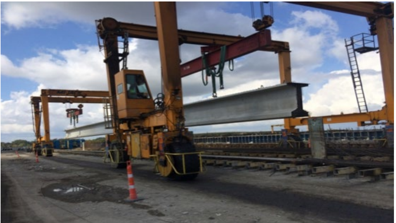
Figure 6. Typical prestressed bridge beam being fabricated at Valley Prestress Products
