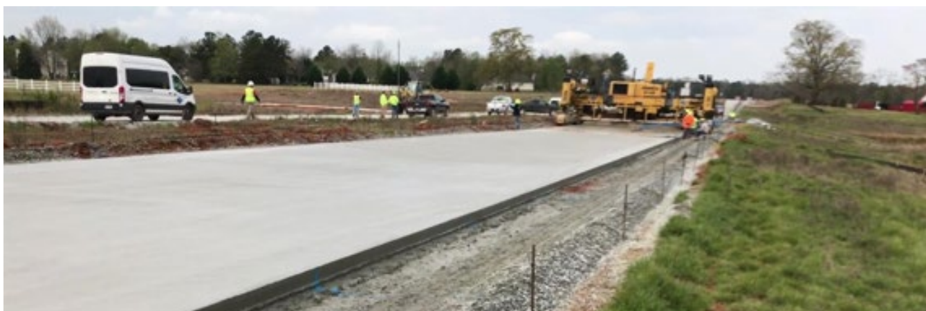
Figure 5. Completed section of highway with added EdenCrete
