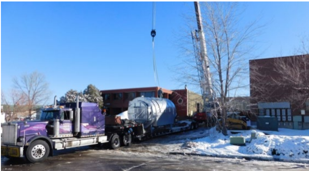
Figure 1. Reactor Being Lifted off Low Loader.
