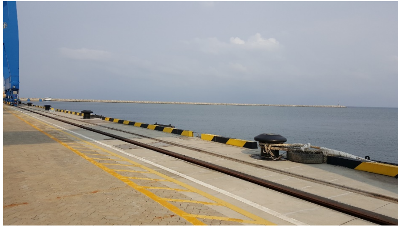
Figure 2: Ship berthing area at the Kribi Port suitable for Panamax size vessels, with breakwater in the distance
