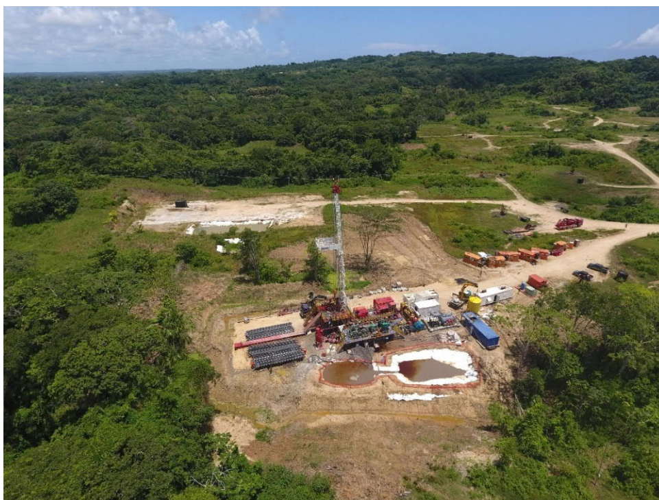
Drilling operations at Morne Diablo field
