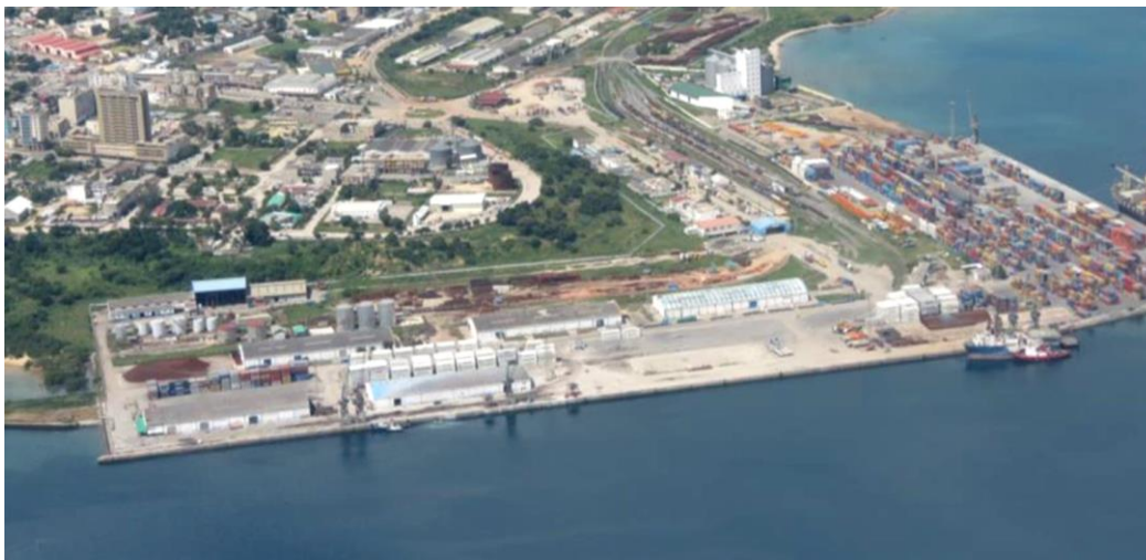
Figure 2: Container storage and loading facilities at the port of Nacala
