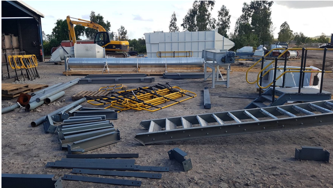
Figure 3: MDS installation underway.
