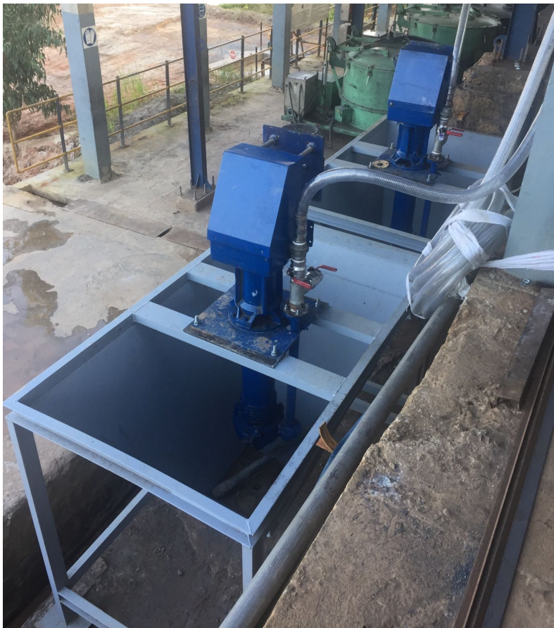
Figure 2: Completed flotation recycle bins installed.
