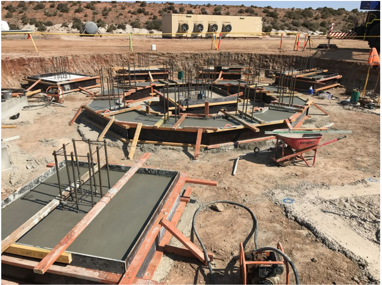
Figure 4 | Concrete works for Thickener
