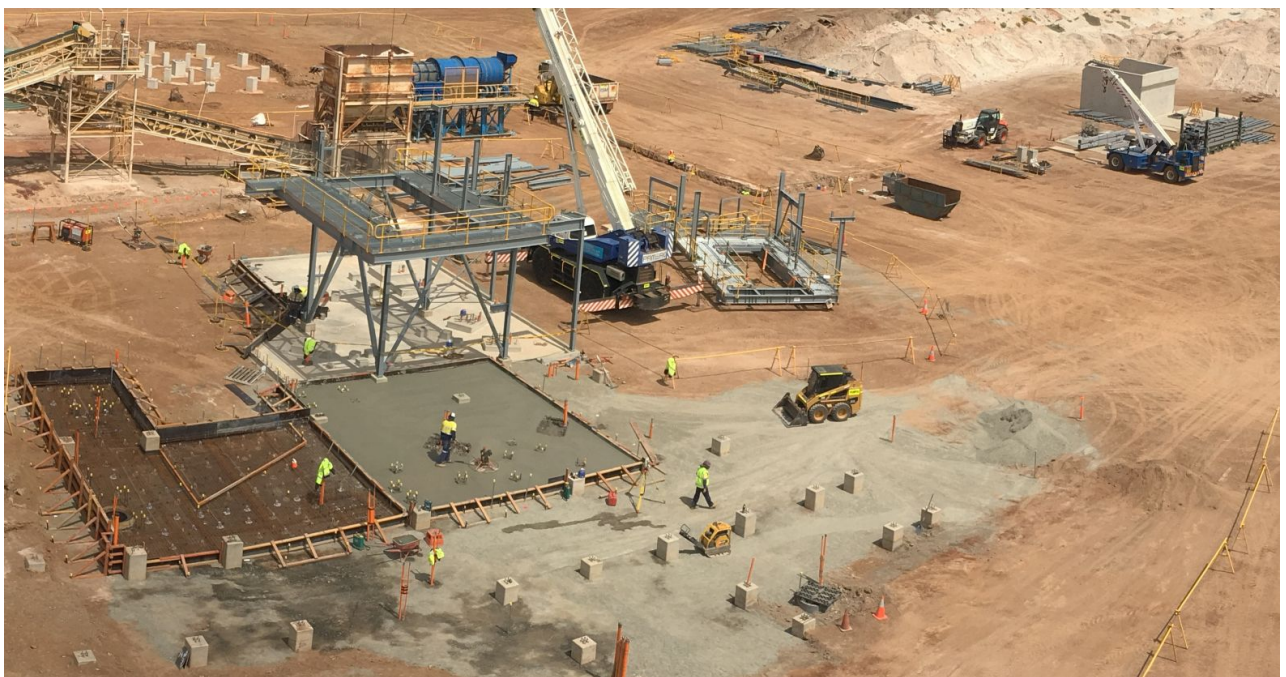
Figure 5 | Feed Bin Wall & Concrete Footings completed
