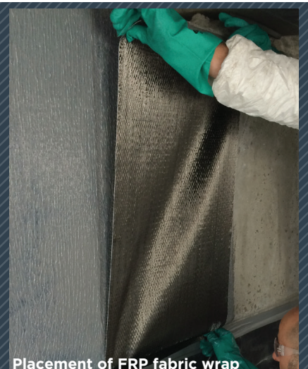
Placement of FRP fabric wrap
