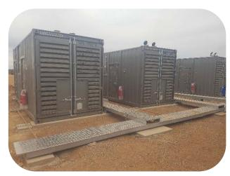
The 6.5MW diesel-fired power station at Pantoro Resources Halls Creek Mine (right).
