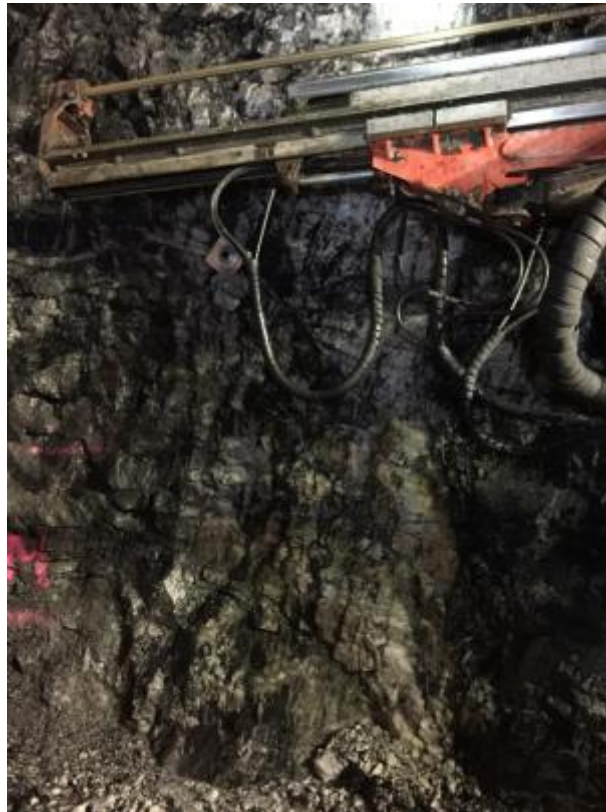
Figure 2: Photograph of the first development to intersect the Alliance South shear. 1060 Cross cut developed due East from the Decline (30m to the right of picture) to intersect the Shear at 90 degrees
