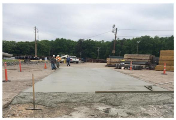
Figure 2. Partially poured slab showing minimal sub-base preparation
