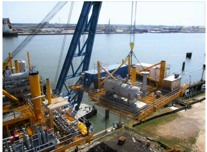
Stacking of Cellar deck.
