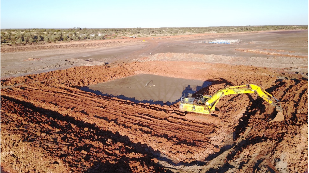
Figure 7: Construction of an Evaporation Pond at Lake Wells
