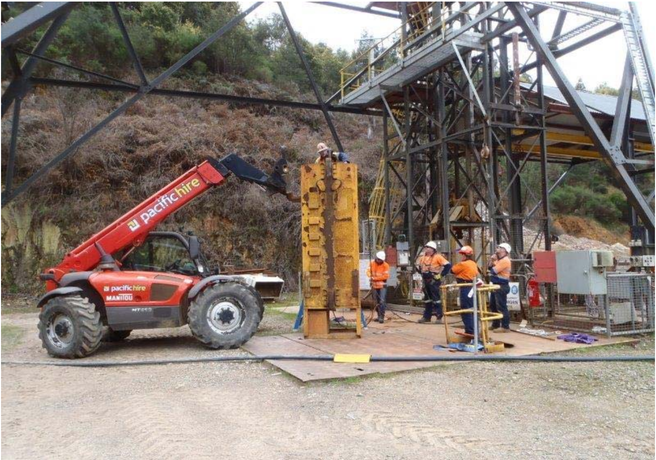
Photo 1 Shaft conveyance removed for Non Destructives Testing (NDT) and painting as part of shaft compliance and winder commissioning.
