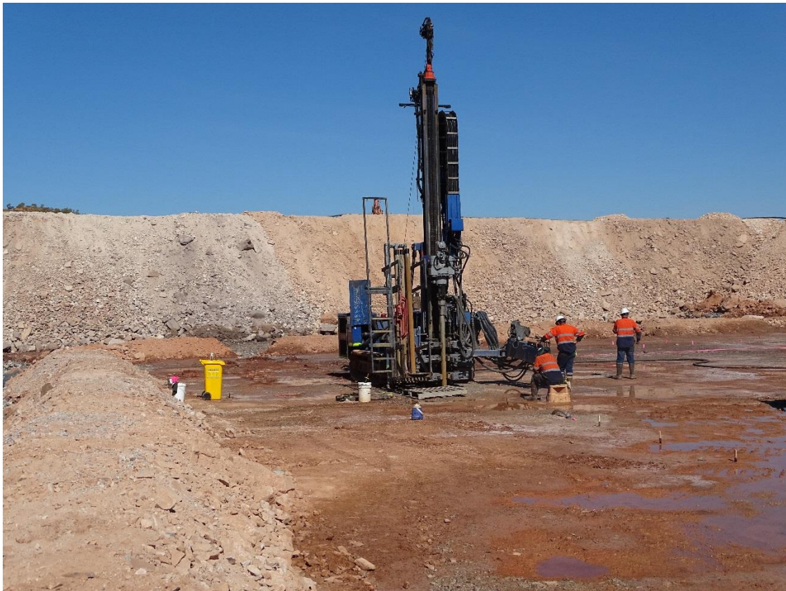
Figure 8: Drilling vertical drains – 29 August 2017
