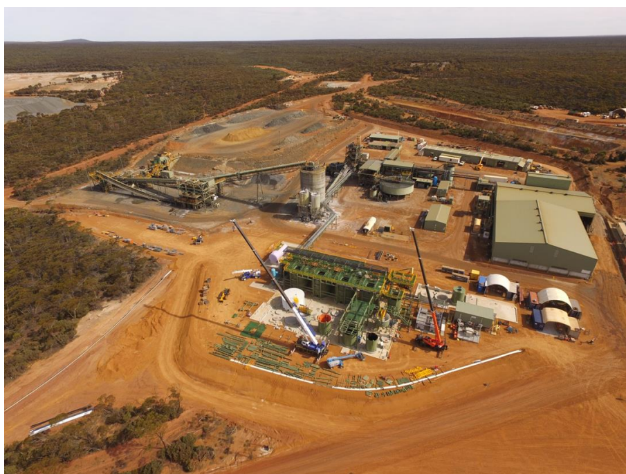
MREP construction in foreground of the Cosmic Boy Concentrator
