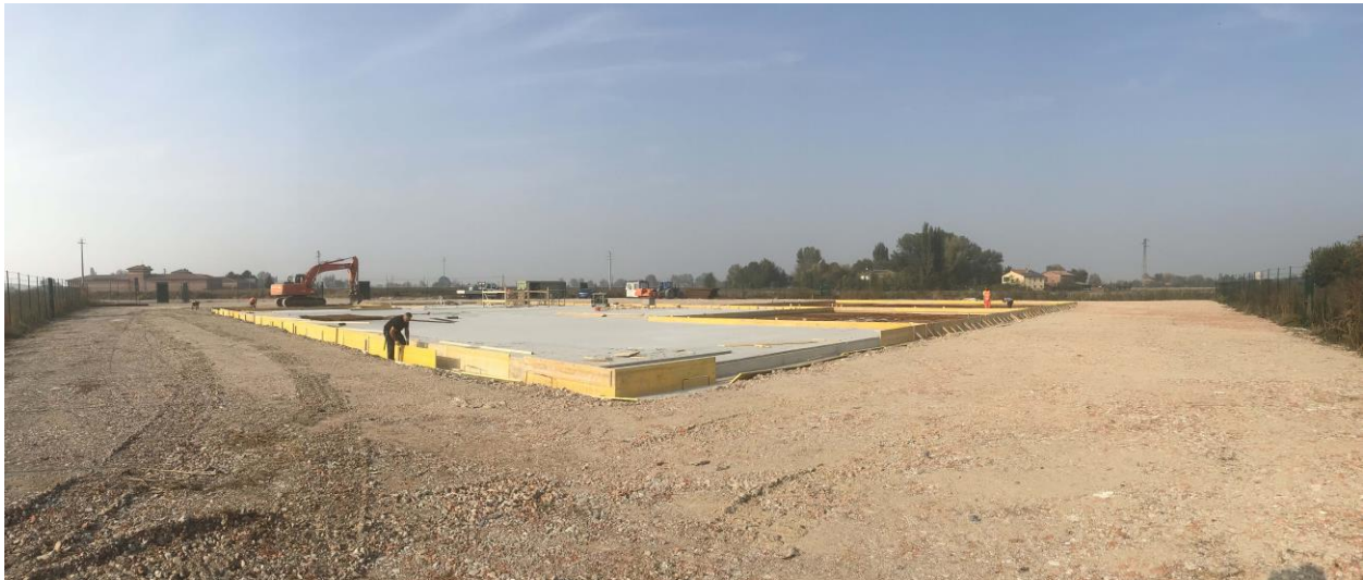
1 Civil works at Podere Maiar1dir well
