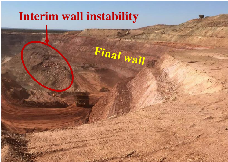
Photo 2: M4 Southern end looking north digging to 1055mRL
