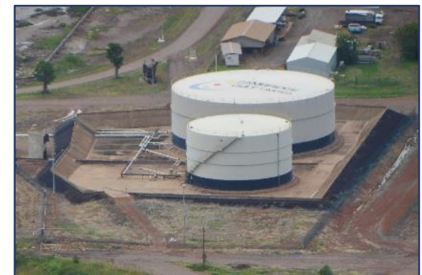
Wyndham Tank 10 (at rear)
