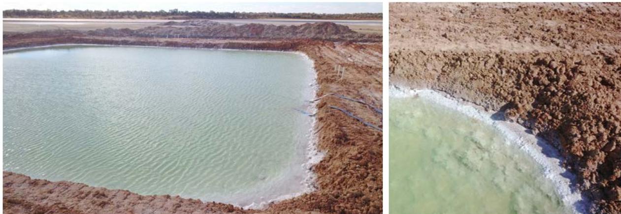
Figure 3: Pond 3 Constructed with Salt already forming
