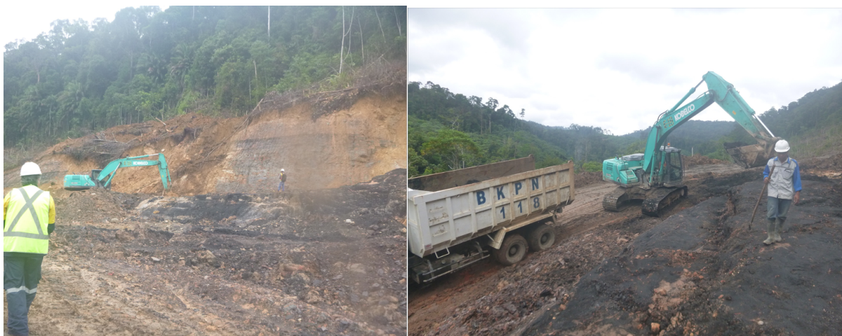
OB Removal and coal cleaning at BBM-Anak Project
