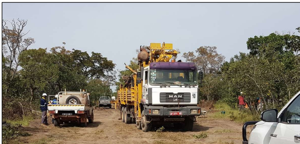
Figure 2: Preparing to drill, Yando
