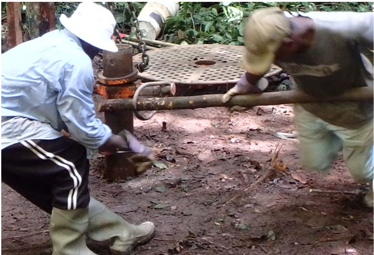
Image 3: Banka Drilling in operation.
