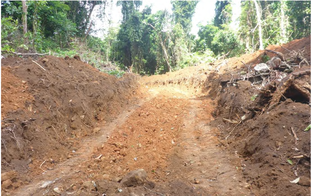
Image 2: Trench 4 prior to commencing deeper excavation.
