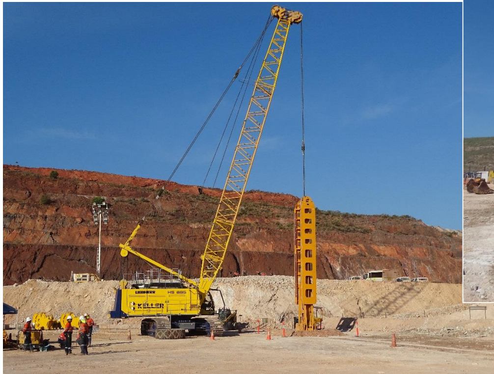
Specialised excavator digging pilot seepage barrier panel, September 2017.
