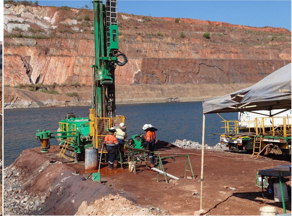
Drilling to install seawall monitoring instrumentation, October 2017.
