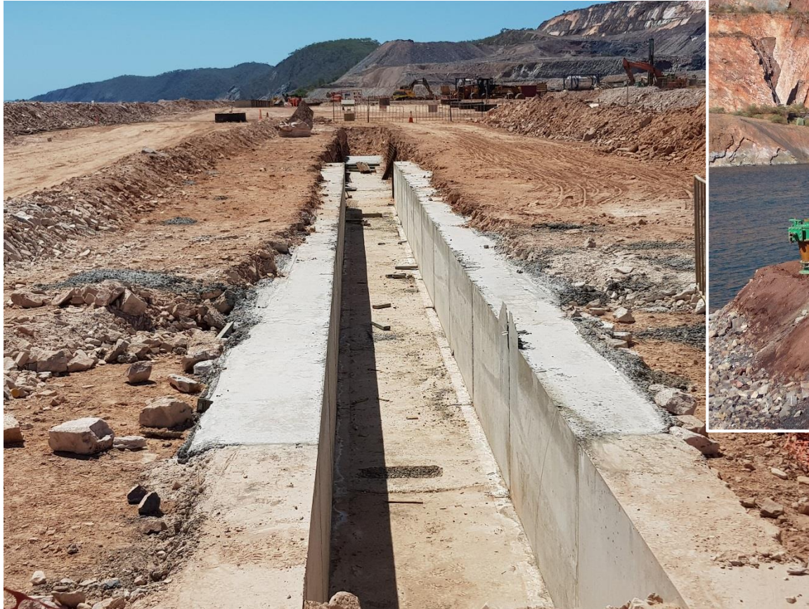
Seepage barrier guide wall construction, October 2017.
