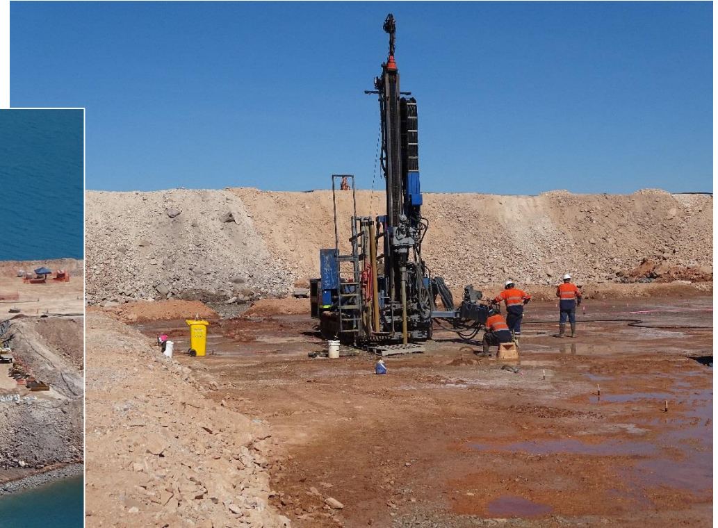
Drilling vertical drains, August 2017.
