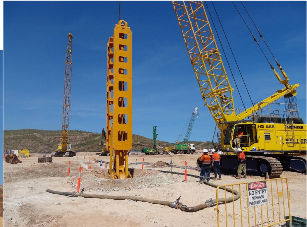
Excavation of pilot seepage barrier panel, September 2017.
