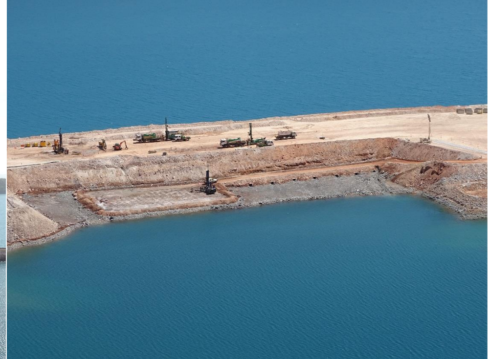
Grouting holes being drilled (upper) and vertical drains being drilled (lower), September 2017.
