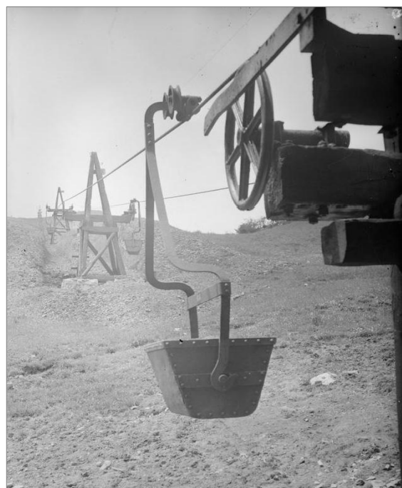
Figures 3 & 4 – Aerial ropeway & ore delivery buckets from La Profunda to Villamanín plant (circa 1924)
