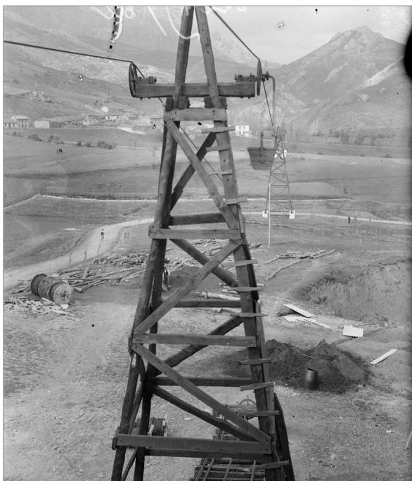
Figures 3 & 4 – Aerial ropeway & ore delivery buckets from La Profunda to Villamanín plant (circa 1924)
