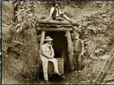
Pictures illustrate the mine entrance and tramway constructed in 1910-11
