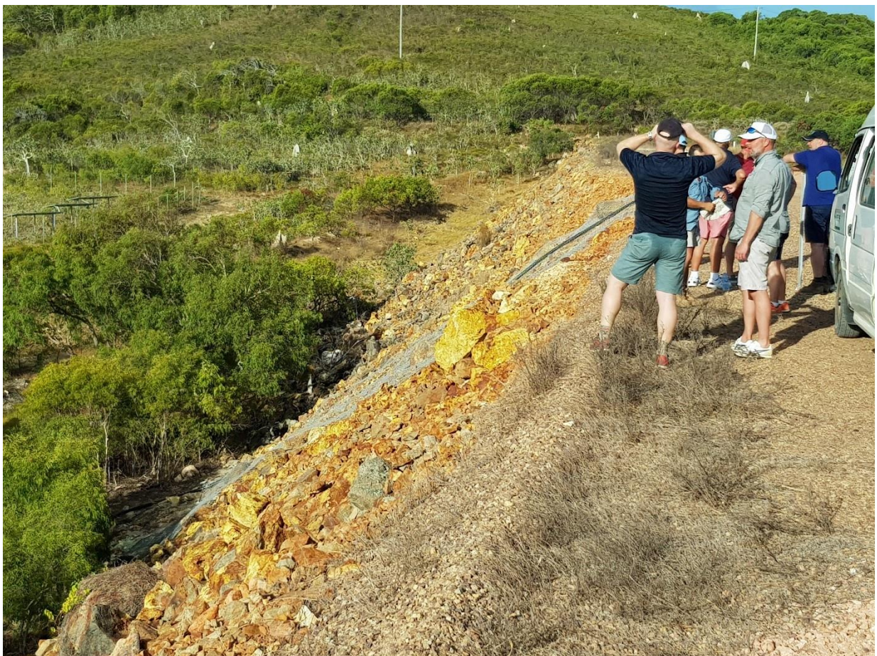
Figure 1. Loose rock construction of the process water dam wall. The yellow and brown stained rocks are related to oxidation of sulphides. High sulphides are often conducive to good gold values.
