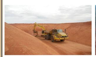
Primary Crusher – Excavation of Raft Foundation
