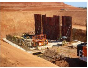
Primary Crusher Raft Foundation (750 m<sup>3</sup> of concrete)
