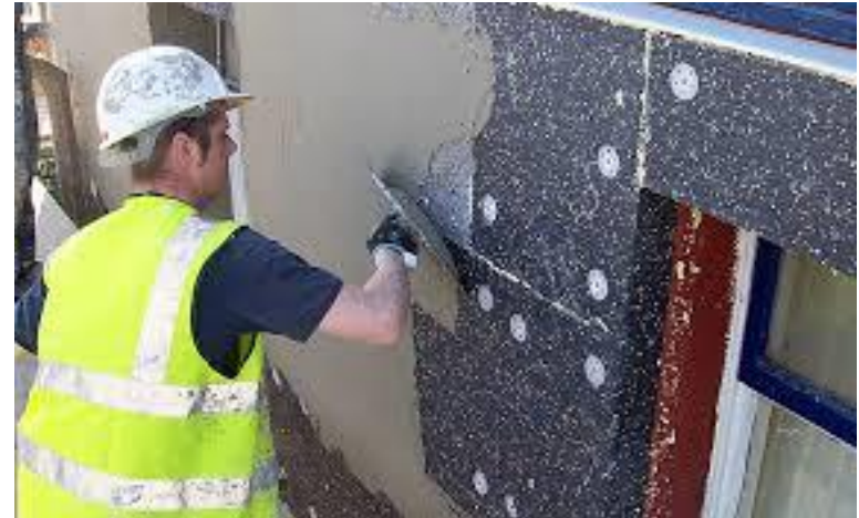
Installing flame retardant insulation foam
