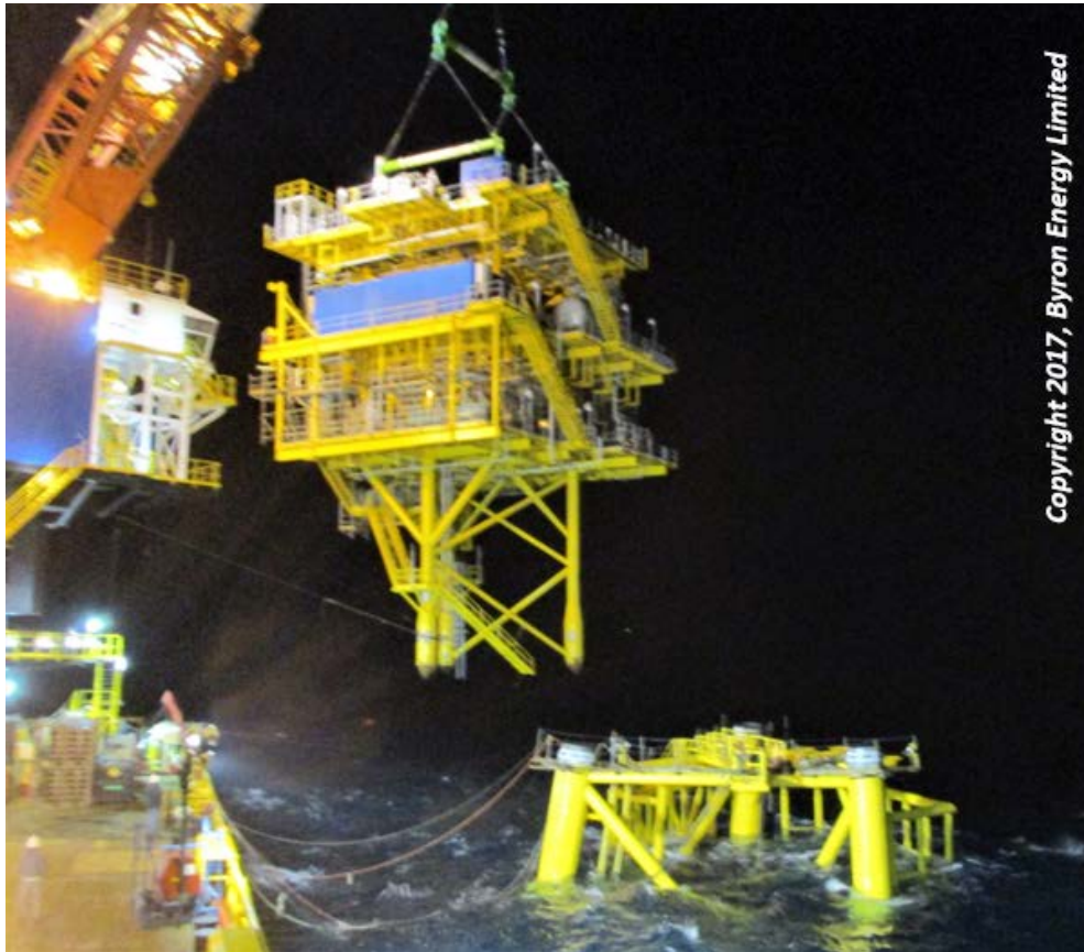
Lifting the SM 71 F Platform decks on to the jacket
